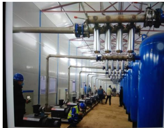
Fig 7: CMVS equipped with MINK Rotary Claw Vacuum Pumps by Busch at Wuhan, China [9]
